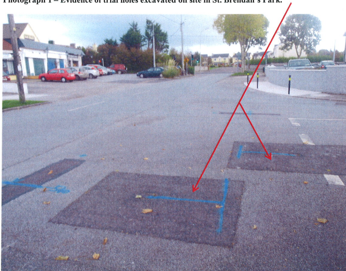
Photograph 1 – Evidence of trial holes excavated on site in St. Brendan's Park.
