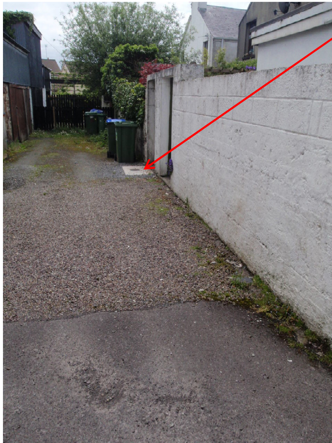
Photograph 3: Cloonmore Road, no visible trench scar, but new meter chambers observed.
