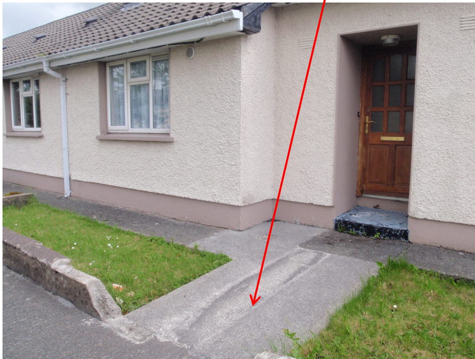
Photograph 1 Balloonagh Close; trench scar to stopcock.
