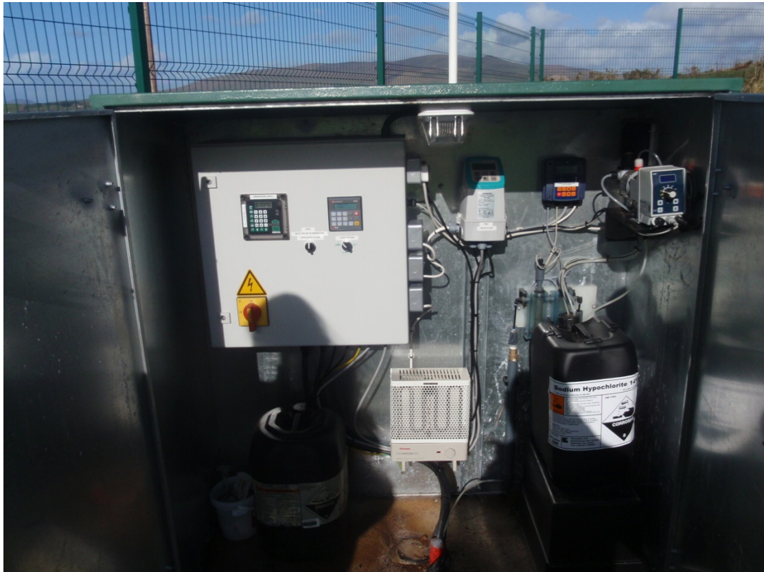
Photograph 1: Duty chlorine dosing pump only at the booster station, no standby dosing pump. The expiration date on the chlorine drum was observed to have passed.
