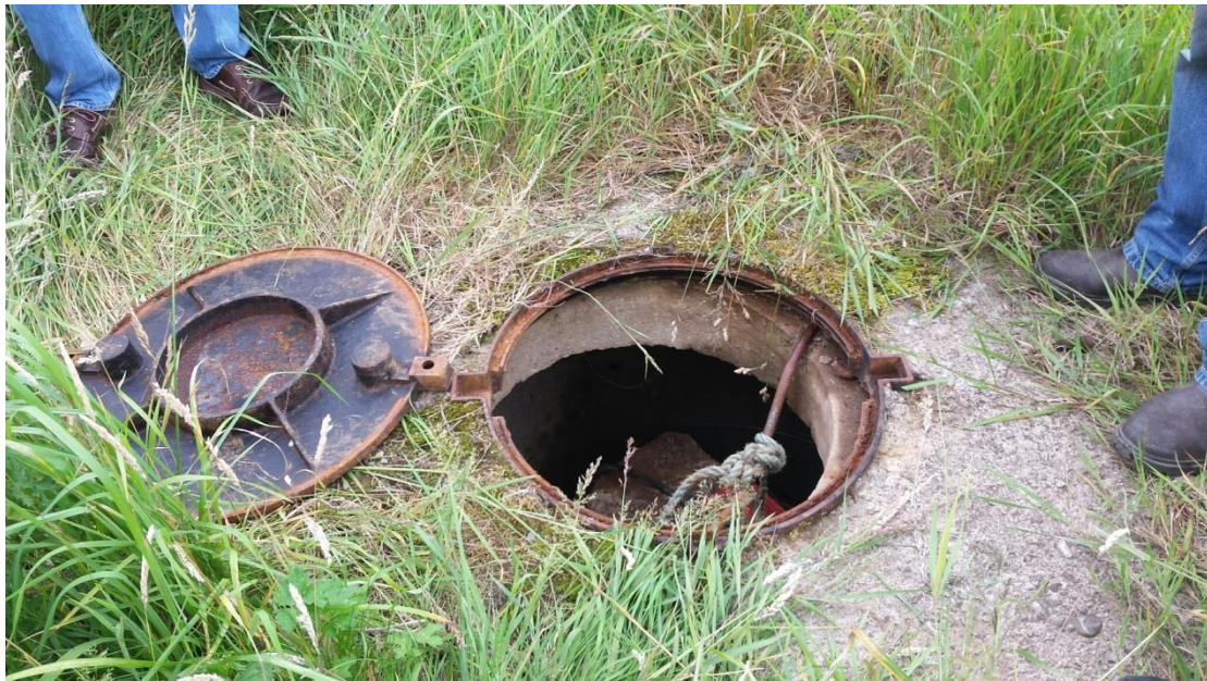
Photograph No. 1: Borehole chamber located below ground level
