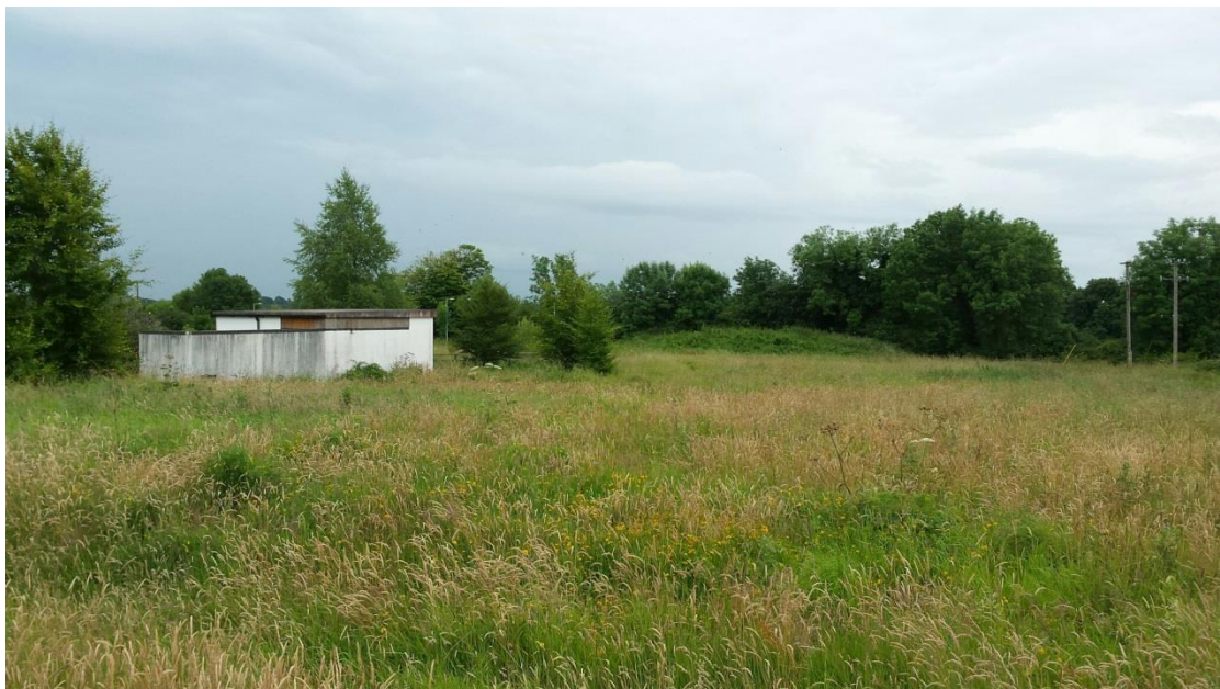
Photograph No. 3: No fencing around borehole or Water Treatment Plant.
