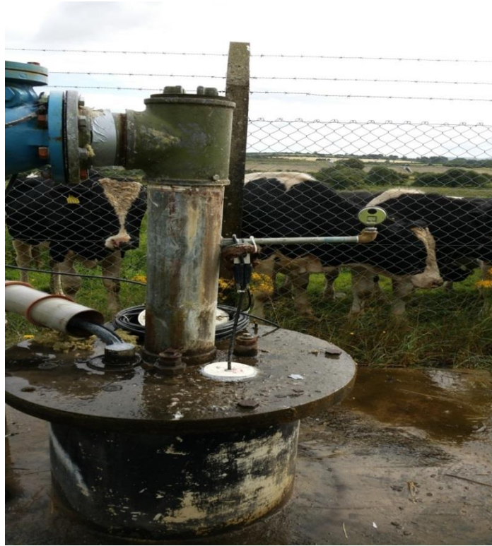
Photograph No. 1: Borehole No. 1 Wellhead Completion with cattle grazing in background (< 3m)
