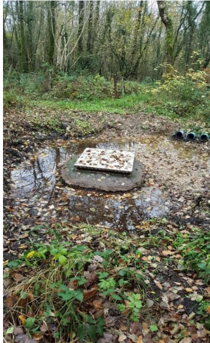
Photo 2 Fill point of fluorosilicic acid day tank
