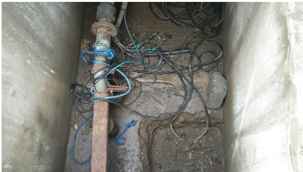
Photo 2: Redundant Borehole B (Durrow) – not sealed or capped.
