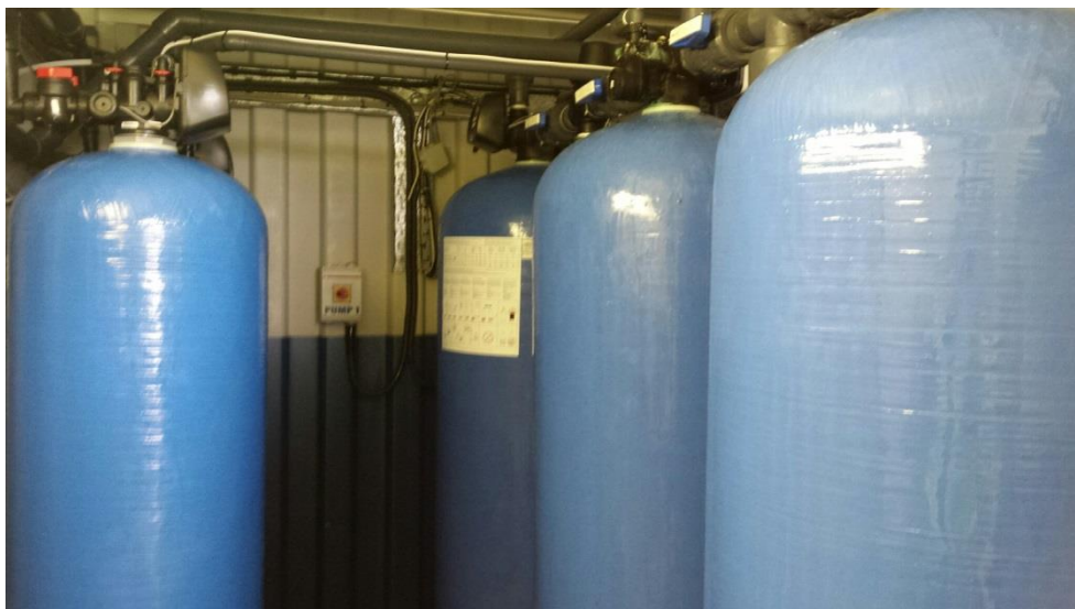
Photo 3: Ion exchange units for nitrate removal at Fermoyle treatment plant.
