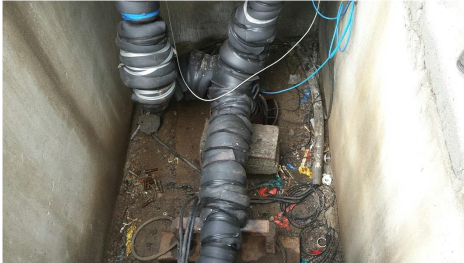
Photo 1: Production Borehole A (Clonking) – not sealed or capped.
