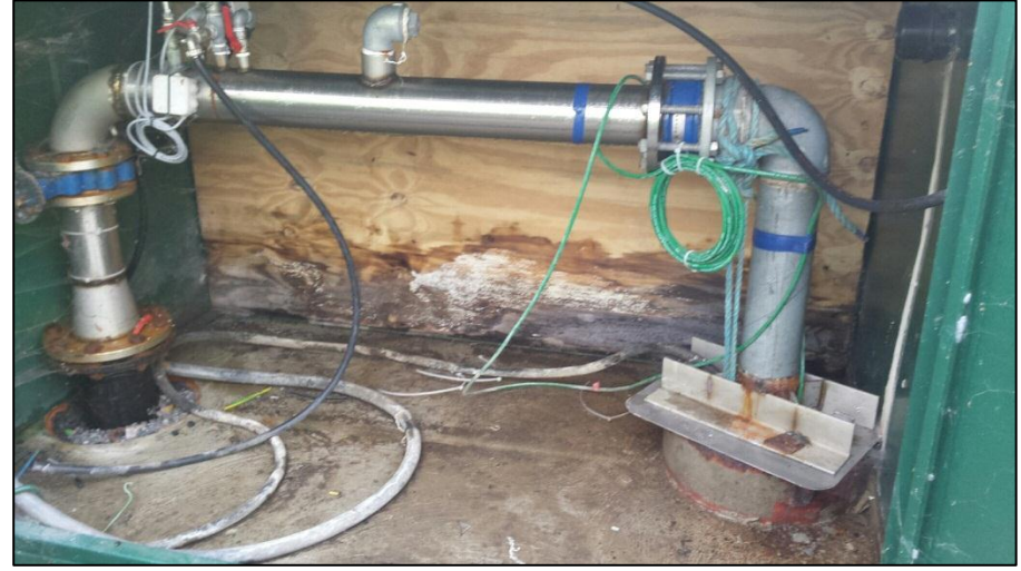
Photo 4: Borehole cover at Eyne No. 3
