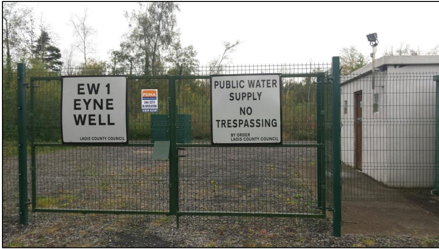
Photo 1: Security compound at Eyne No. 1
