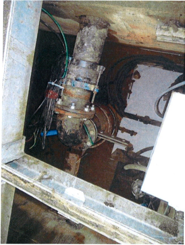
Photograph 1: Standing water in Borehole 2, Derrygarran
