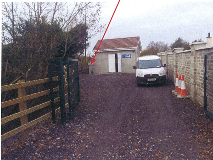
Photograph 3: New chlorination building with sludge holding tank.
