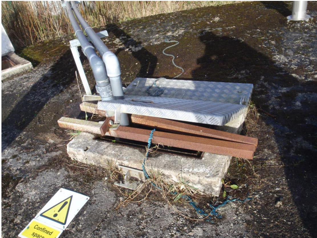
Photograph 1: Inspection hatch at Skagh Spring – cover unable to close to protect spring water from contamination or ingress.
