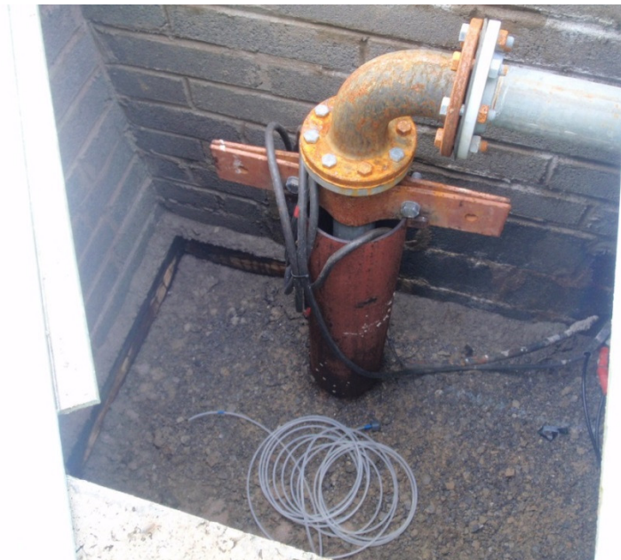
Photograph 2: Top well head above ground level.
