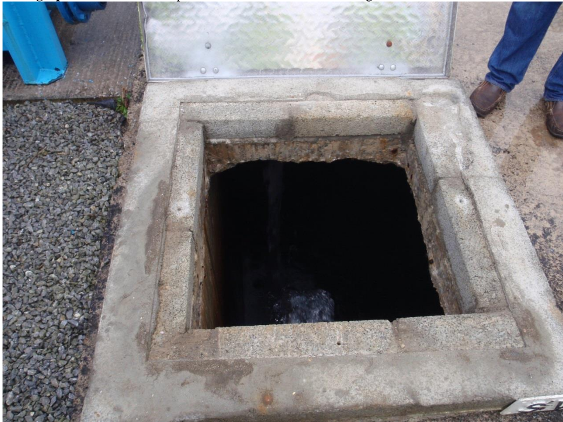
Photograph No. 5 Unsealed inspection hatch to treated water storage tank.
