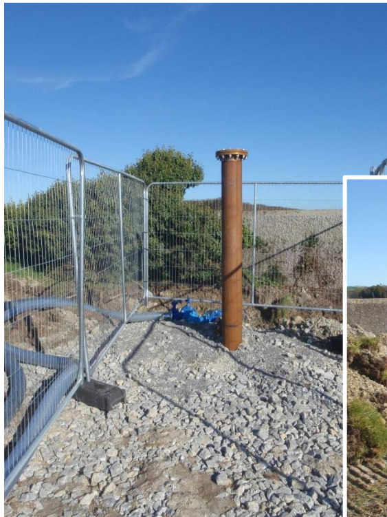
Photograph No. 2a: New trial borehole. To be decommissioned when final production borehole is drilled.
