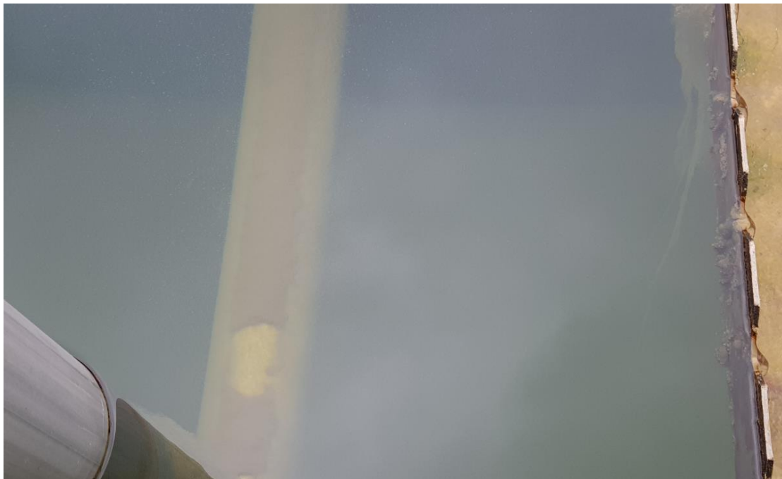
Photo 2 Pin floc evident in clarifer
