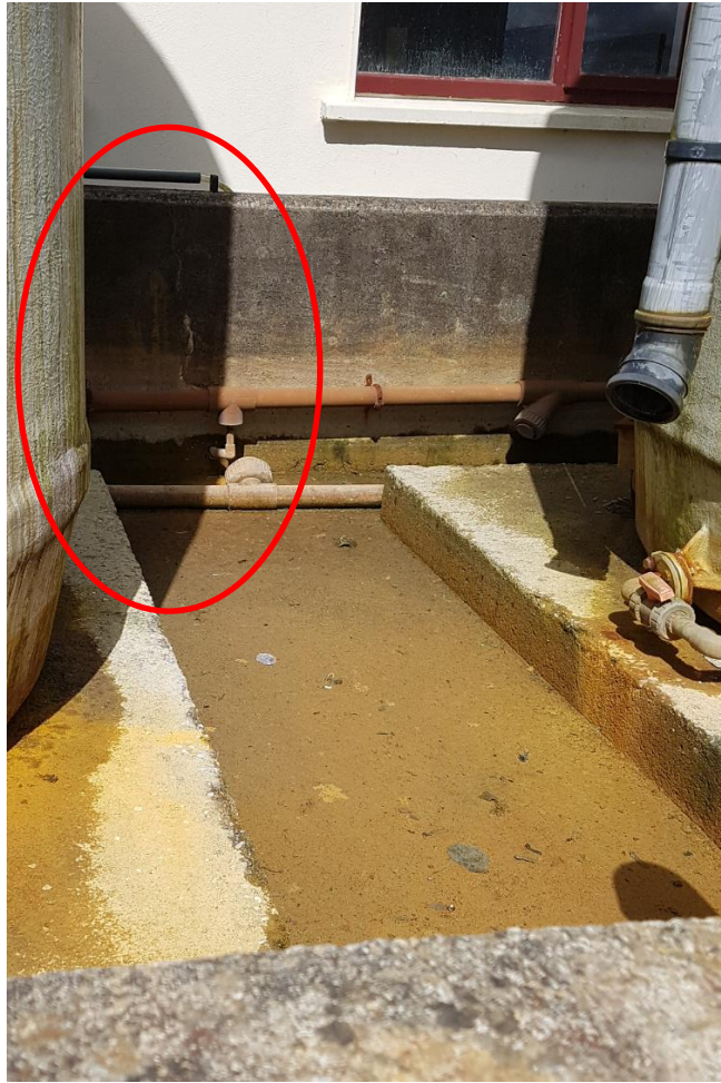
Photo 3 The Chemifloc 101 bund wall appeared to be cracked and had pipework routed through its wall
