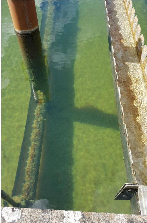
Photo 1 Clarifier pipework rusted and pin floc present
