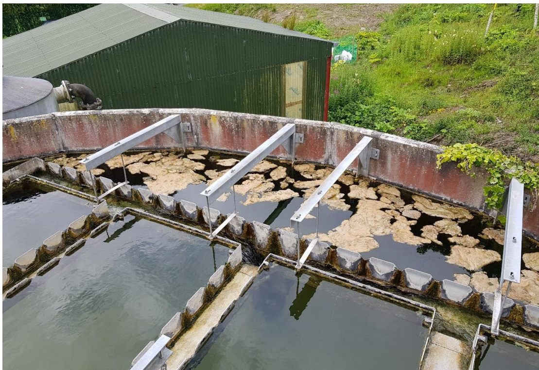
Photo 2. Build-up of sludge/ algal material in New Plant Clarifier and lack of access for cleaning tank and channels. Also shows ivy overhanging the tank edge.
