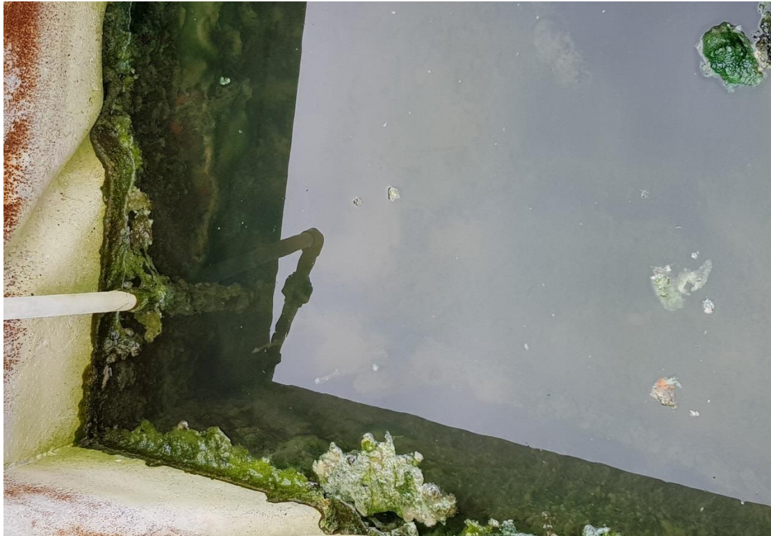
Photo 1. Flocculation tank at Old Plant showing build up of floc/ algal material on tank walls.
