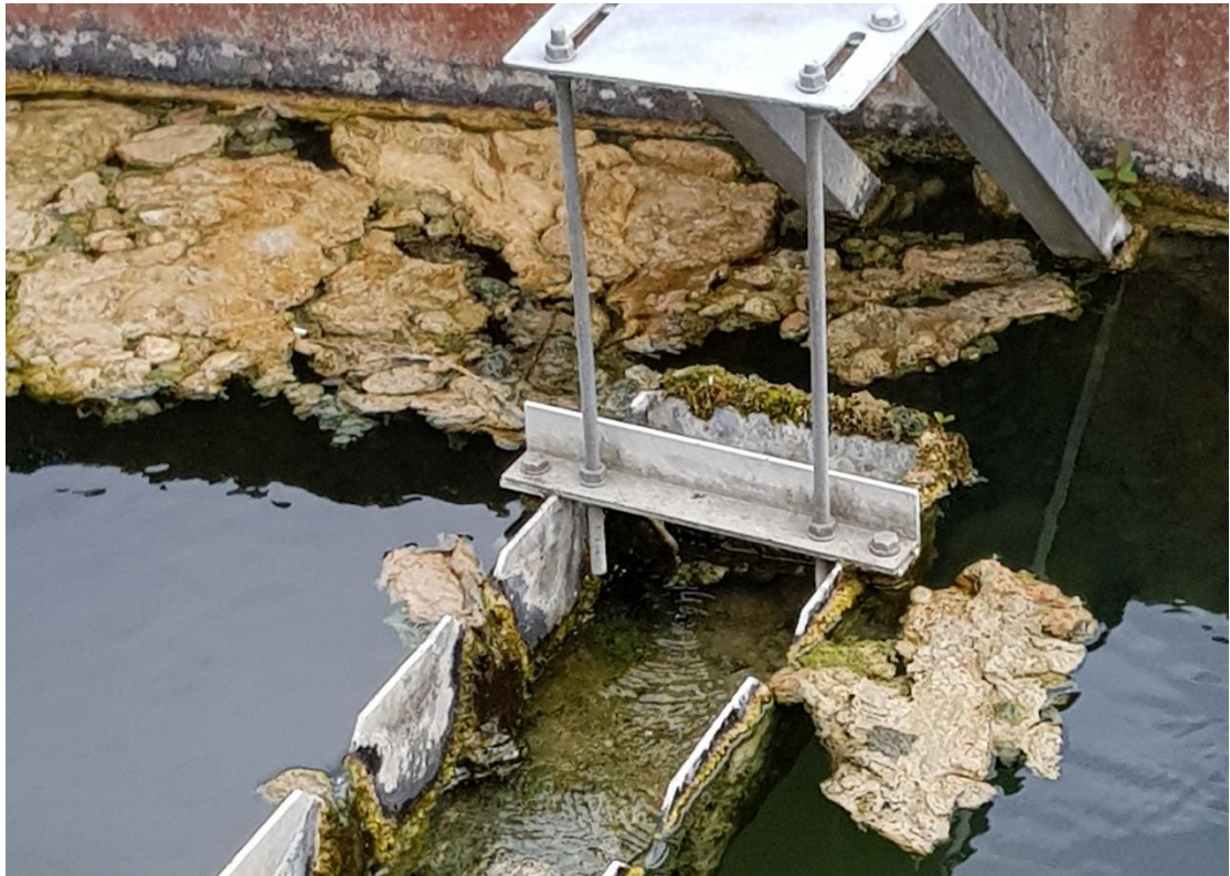
Photo 3. Close up of the sludge/ algal material on water surface and channels at the New Plant clarifier.
