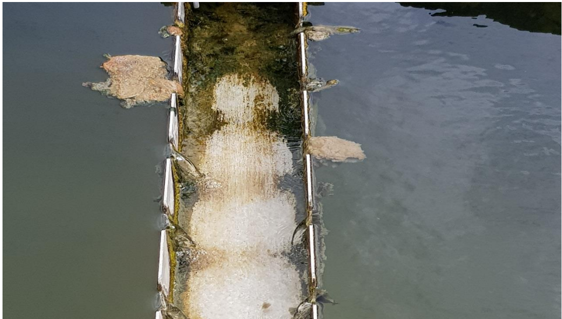
Photo 4. Carryover of sludge/ algal material from New Plant clarifier into settled water decanting channel
