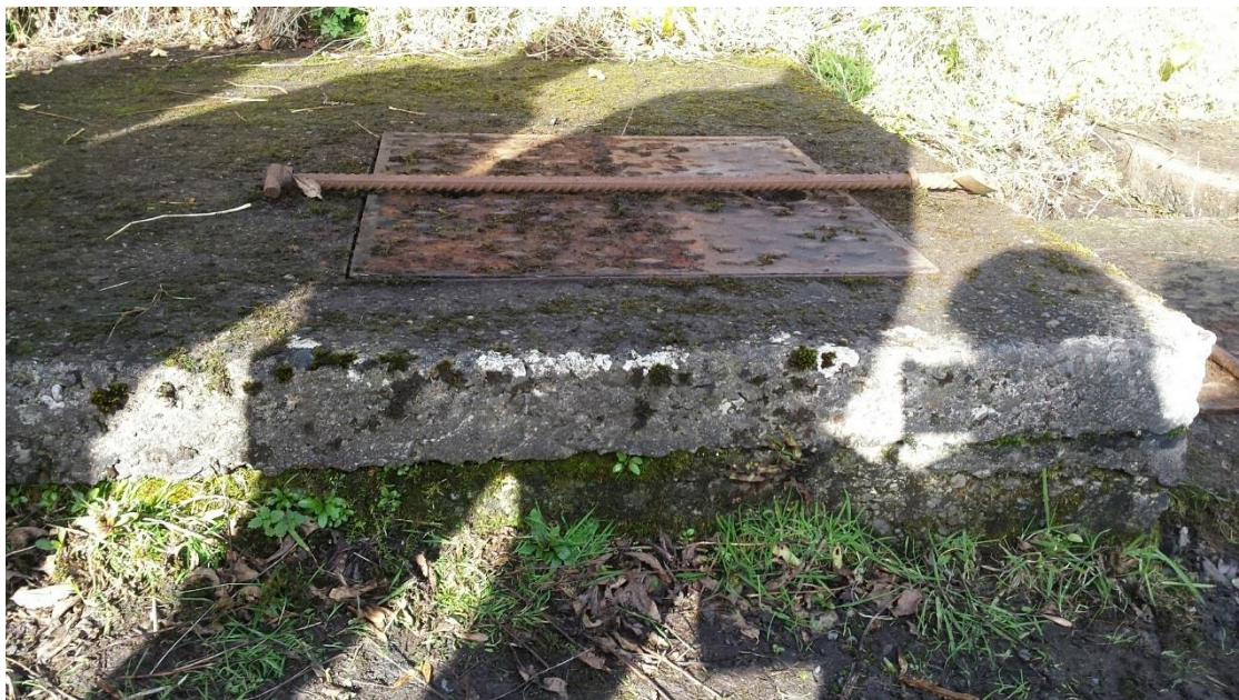
Photo 2: Side of spring chamber showing gap in concrete (potential route of surface water ingress)
