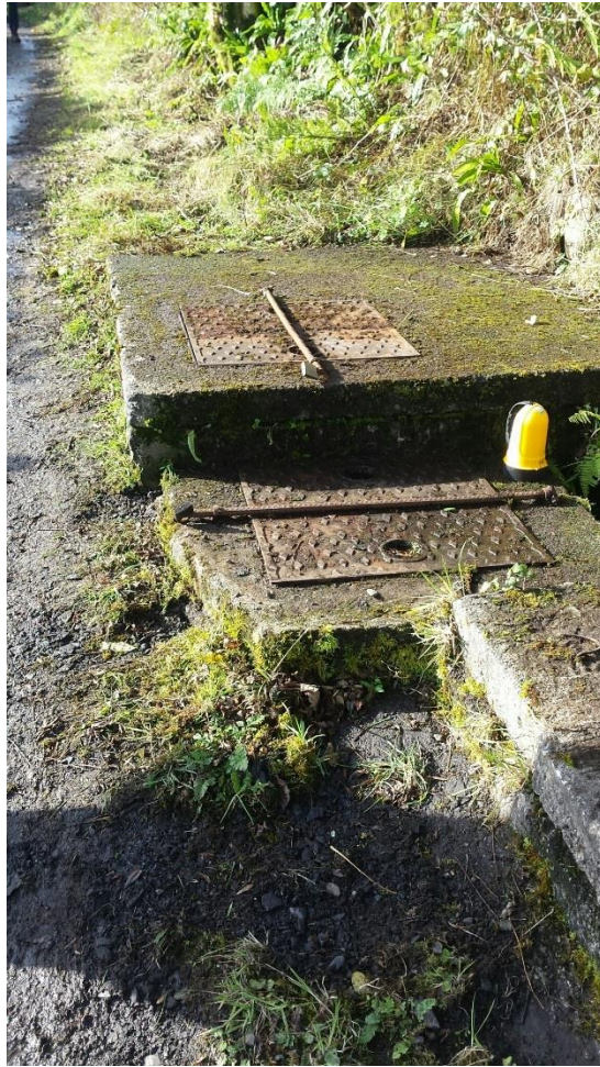
Photo 1: Spring chamber
