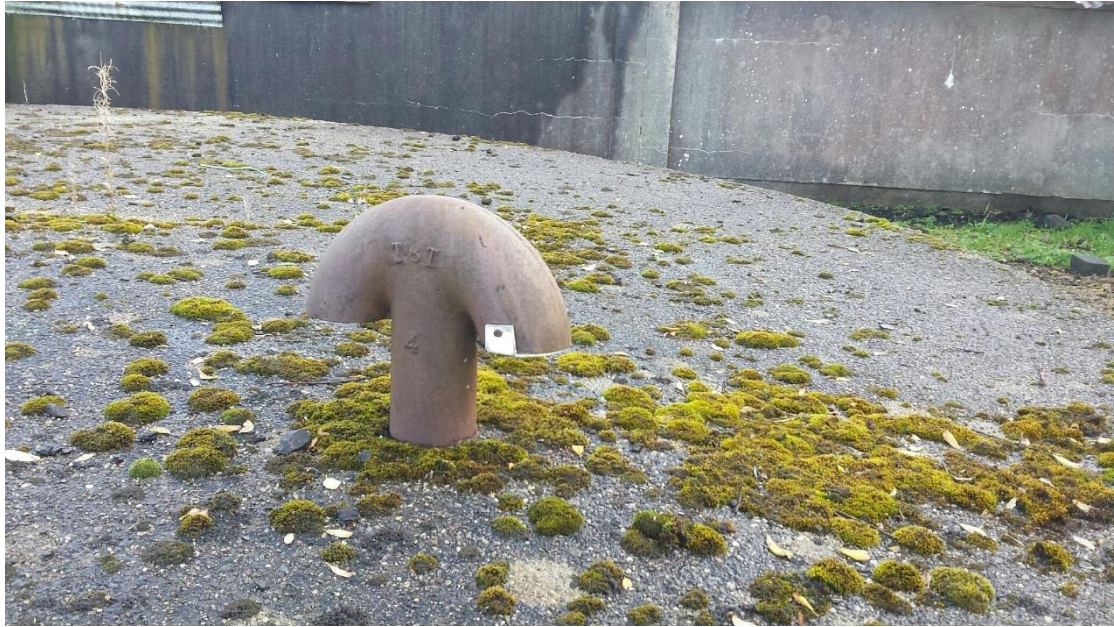
Photo 3: Vent on Town Hall Reservoir – mesh cover missing on one side
