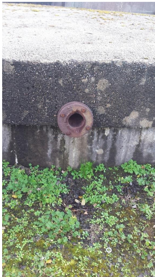
Photo 4: Overflow pipe on Town Hall Reservoir
