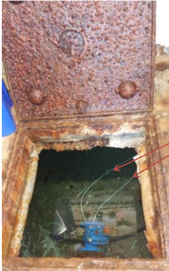
Photo 1 Intake area - containing waste such as black piping, plastic bag and tags and rusted cover.
