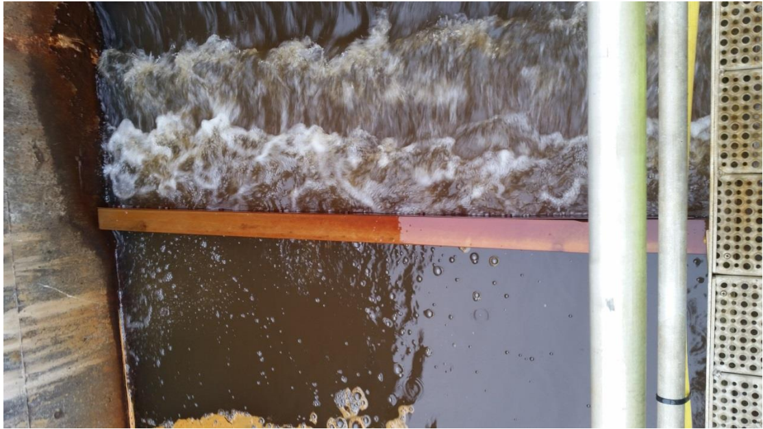
Photo 1. Bar Installed in Chemical Mixing Chamber to Improve Mixing.
