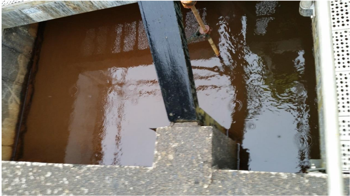
Photo 3. “Dead Zone” in mixing chamber (note sludge build up).
