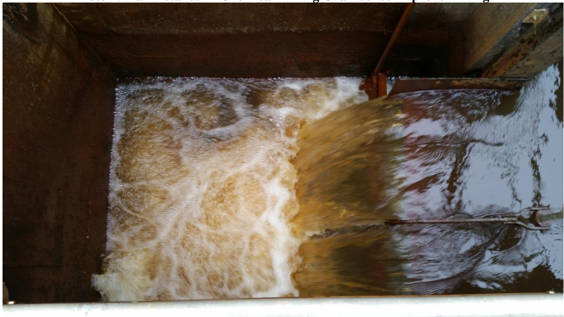
Photo 2. Weir following ferric and poly dosing.
