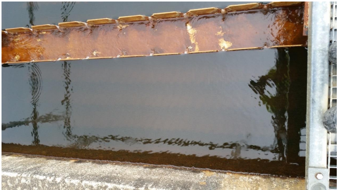
Photo 4. Pin Floc Carryover in Clarifier.
