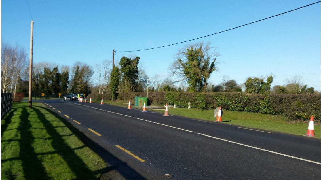
Photograph 1: Location of combined chlorine booster and pump station at Summerhill Road, Dunboyne.
