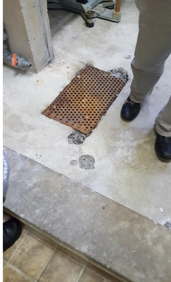
Photograph No. 3: Drainage grate on floor of Hydrofluorosilic Acid Bund
