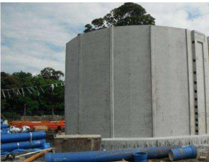
**Photograph 2: Newly constructed raw water blending tank**
