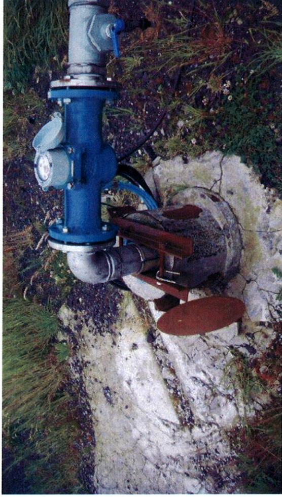
Photograph 3: New borehole at Longford Springs
