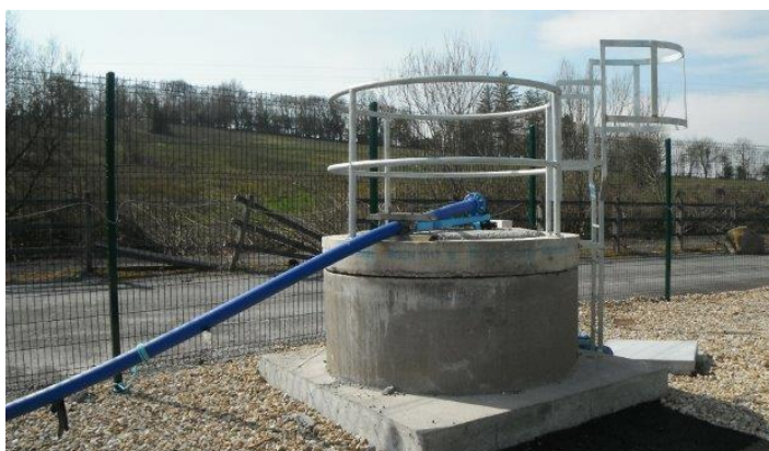
Photograph 1: Borehole that was in operation up until the Cryptosporidium result 0.005/10L was received on 9 th April 2015.
