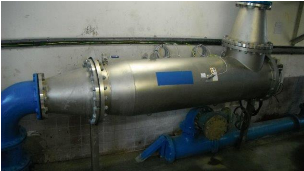
Photograph 1: Xylem/Wedeco Spectrum 900e UV reactor.
