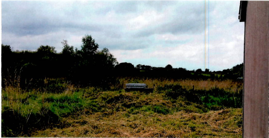
Photo 1 Heapstown Spring Source with protection cover in place (disinfection & pump house on RHS of photo)
