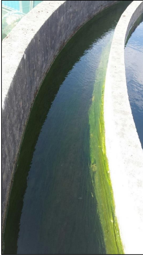
Photo 3: Algal growth on outlet channel in clarifier
