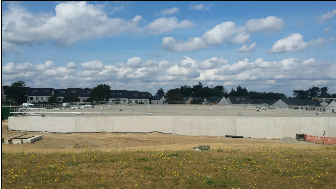
Photo 1: New covered storage reservoir at Ballyboden water treatment plant
