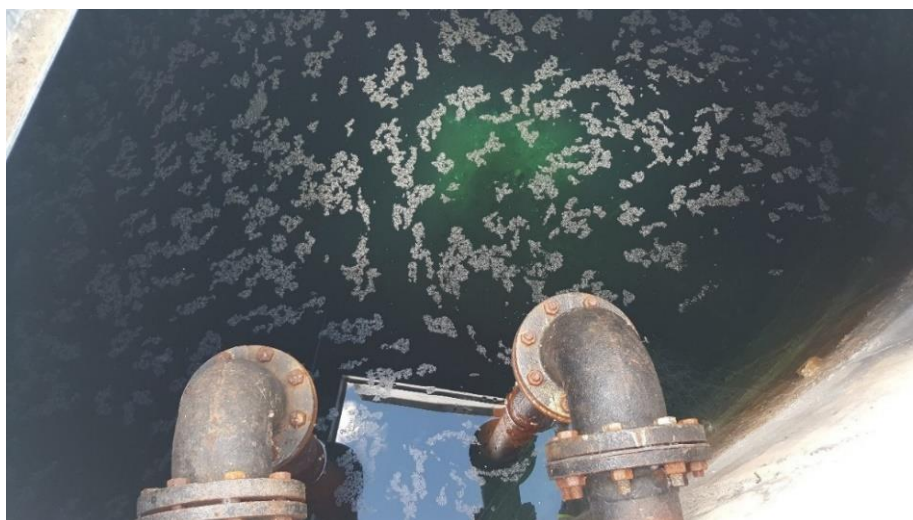
Photograph No. 1: Floating debris visible inside covered collection chamber
