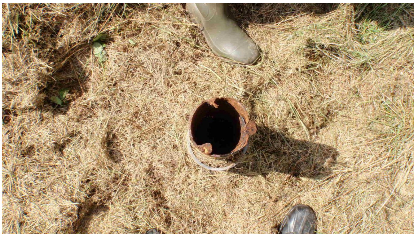
Photograph 1: Damaged vent on reservoir
