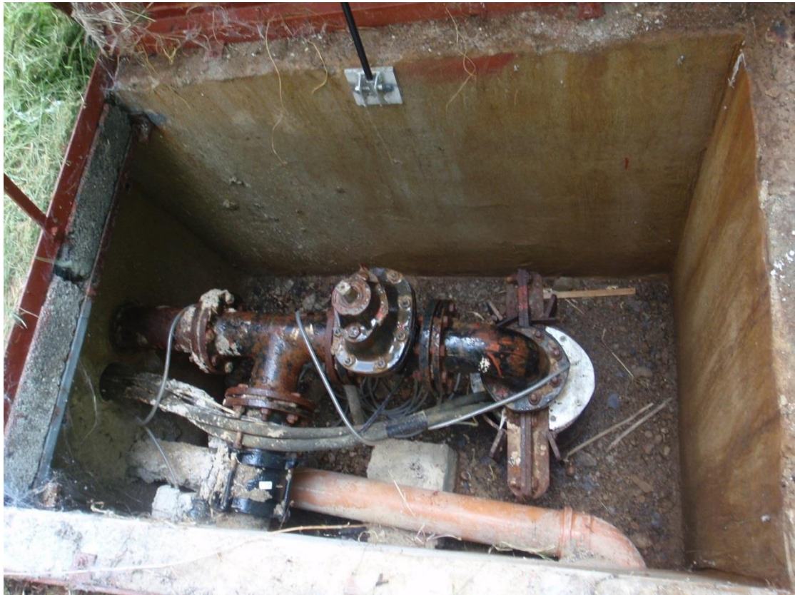
Photograph No. 1: Well Head Completion
