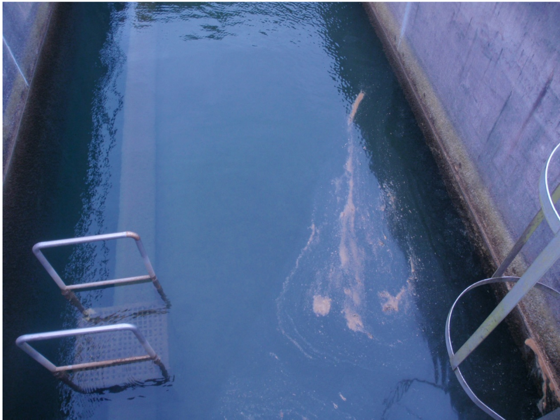
Photograph 5: Appearance of aluminium carry over on water surface in the filter.
