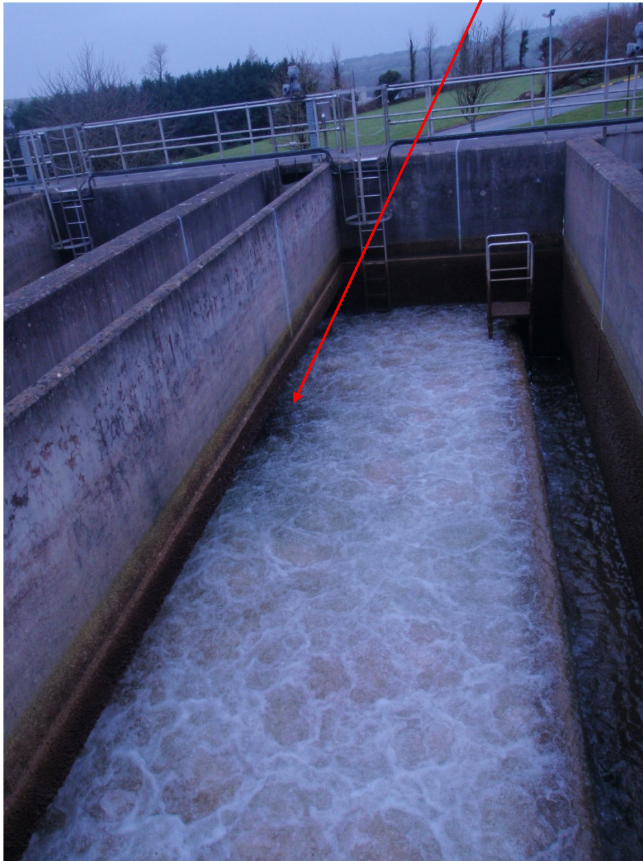
Photograph 3: Dead spot noted during filter no. 3 back wash cycle.
