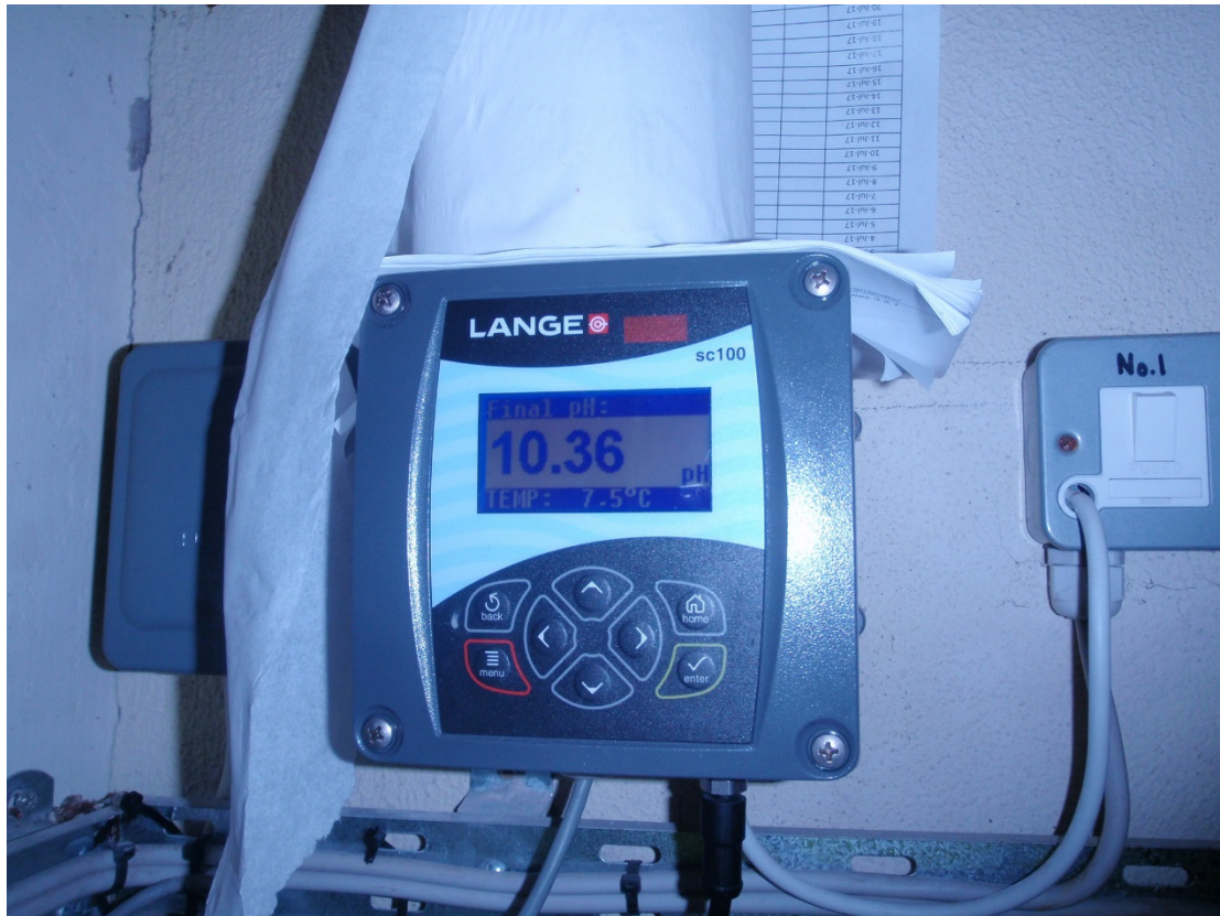
Photograph 6: pH monitor reading 10.36 in the final water.
