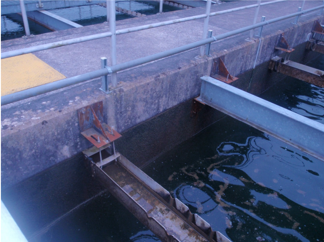
Photograph 2: Scum noted on surface of clarifier and algae noted in decanting channels.
