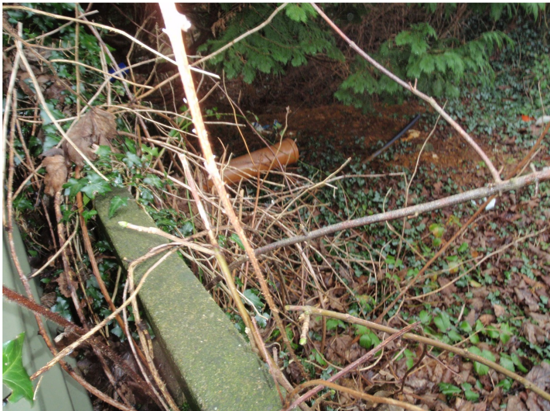
Photograph 2: Outfall pipe from arsenic filter, potential access for vermin.
