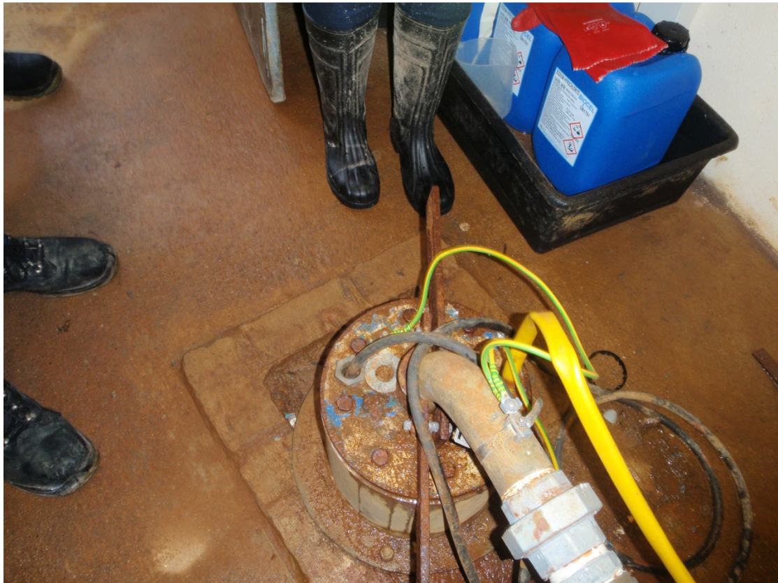
Photograph 1: Capped borehole in the treatment plant.
