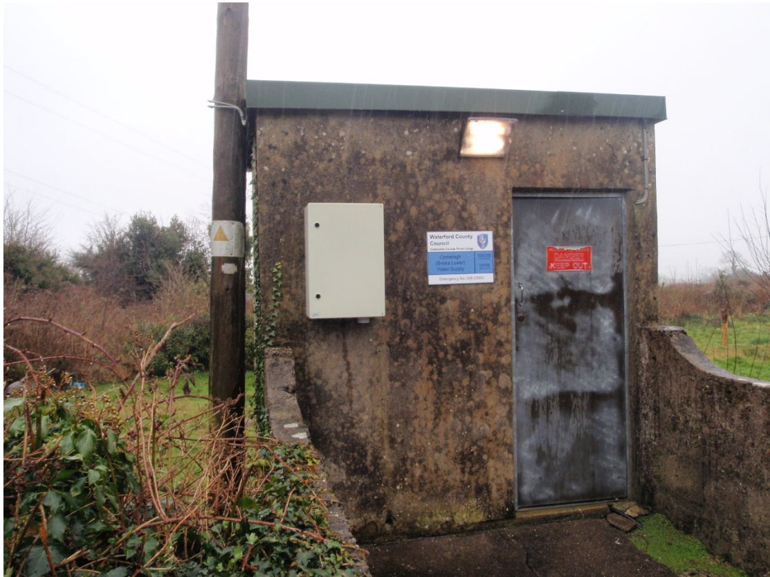
Photograph 1: Comeragh (Briska Lower) WTP.
