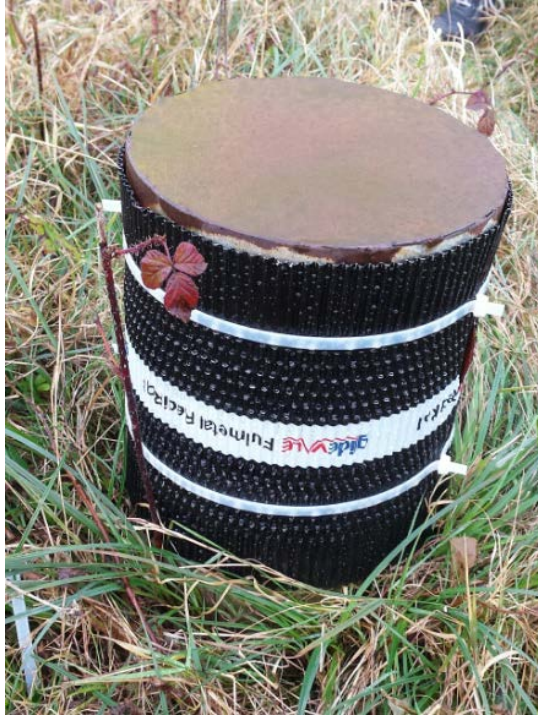
Photo 2 Temporary mesh on Coosan Reservoir vent
