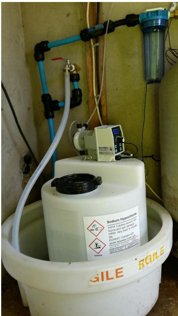
Photograph 2: Bunded day tank and single dosing pump
