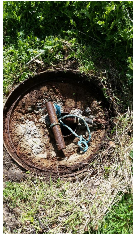
Photograph 2: Wellhead of northern borehole
