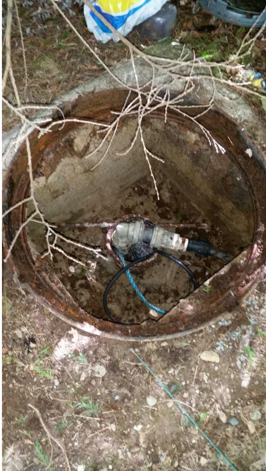
Photograph 1: Wellhead of eastern borehole
