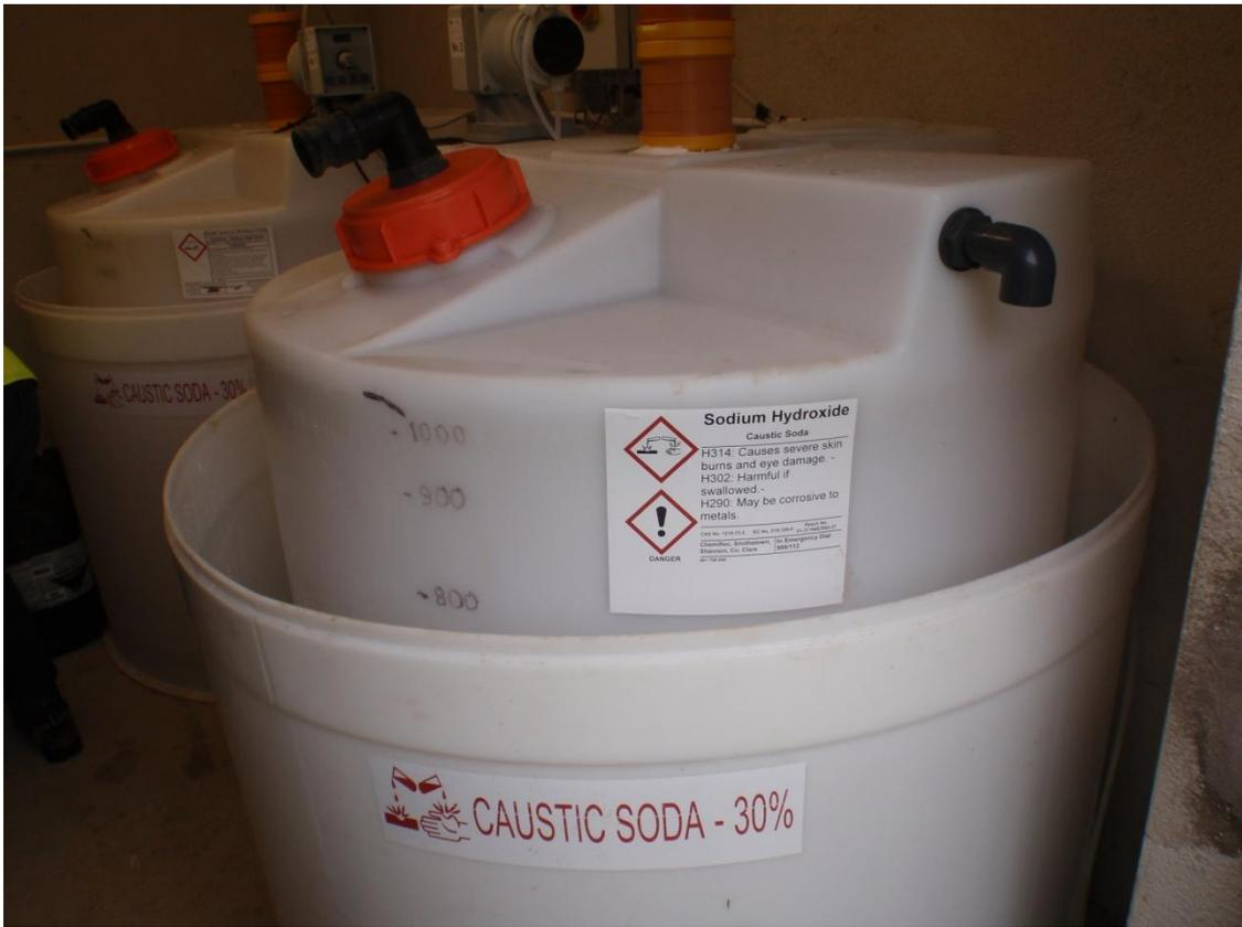
Photograph 1: Caustic soda dosing tanks
