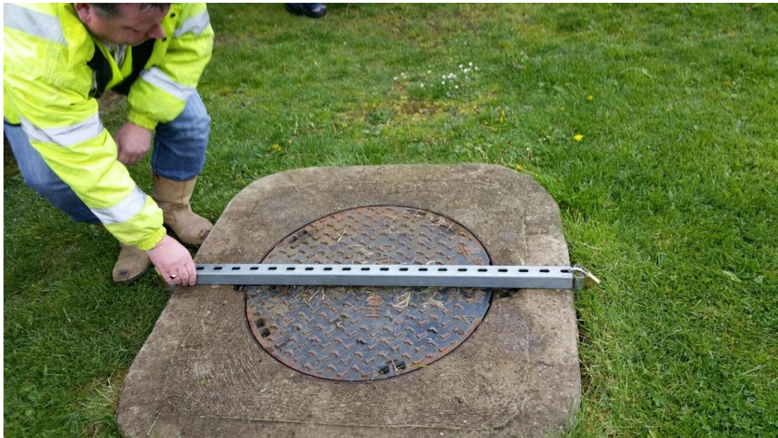
Photograph 2: Borehole cover with lock in place
