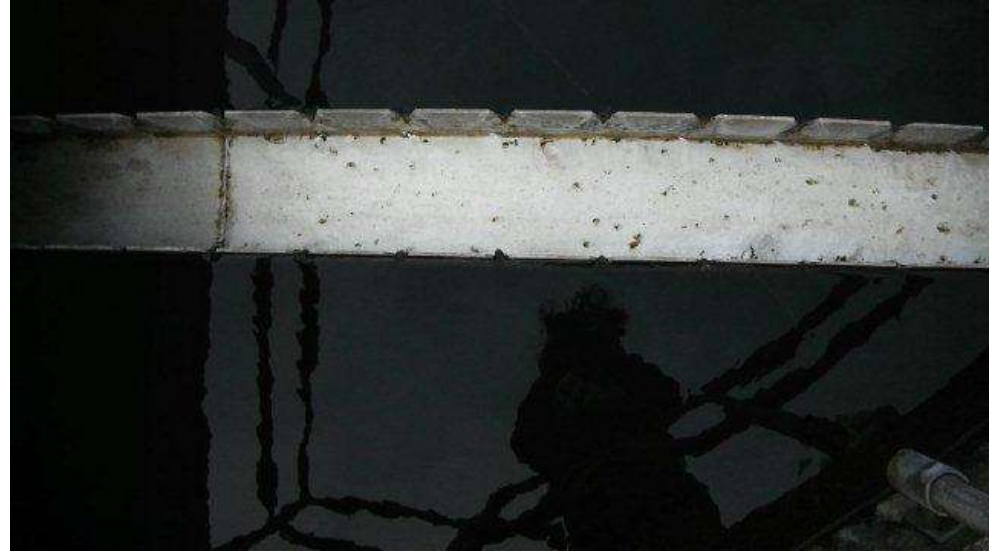
Photograph 2: Holes in the clarifier channel
