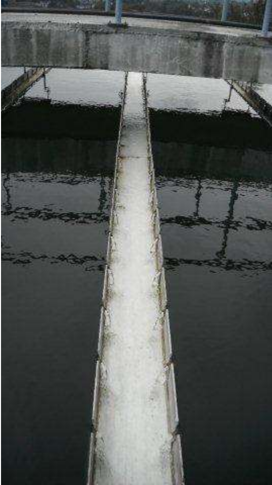
Photograph 1: Uneven flow in clarifier channels
