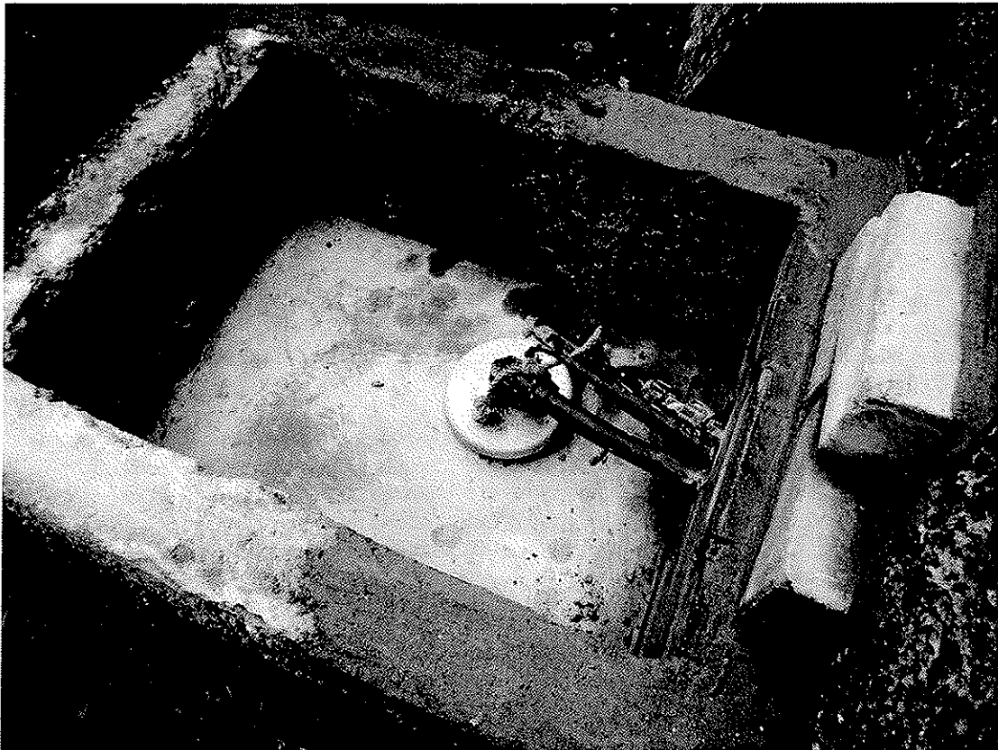
Photograph: Sealed wellhead in an unsecured concrete chamber.
