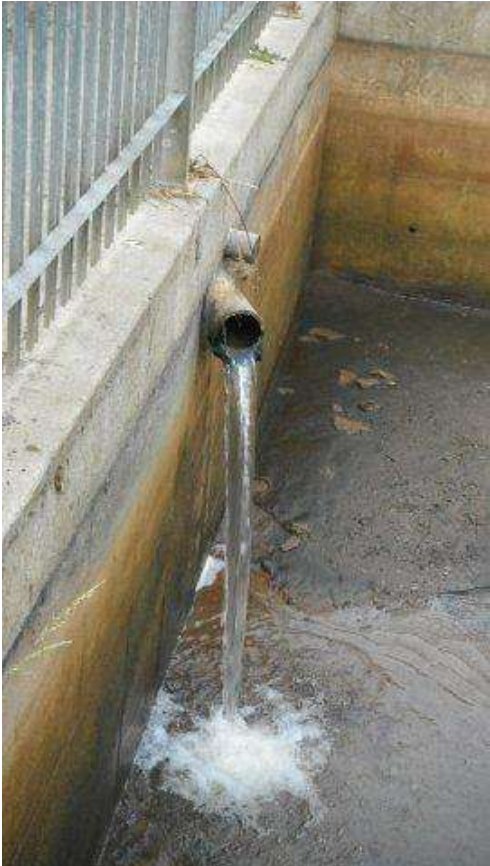
Photograph 2: Clear water from sludge bleeds
