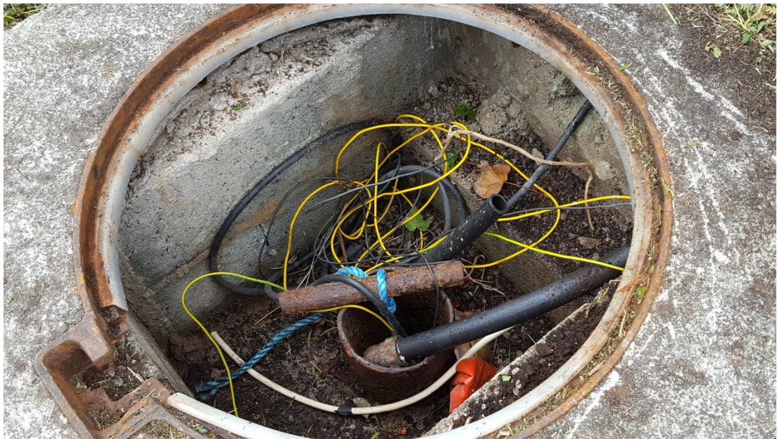
Photograph 2: Brittas Bay North Borehole
