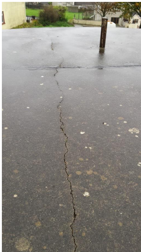
Photo 2. Crack observed in the roof of the Ballyneerin Reservoir.
