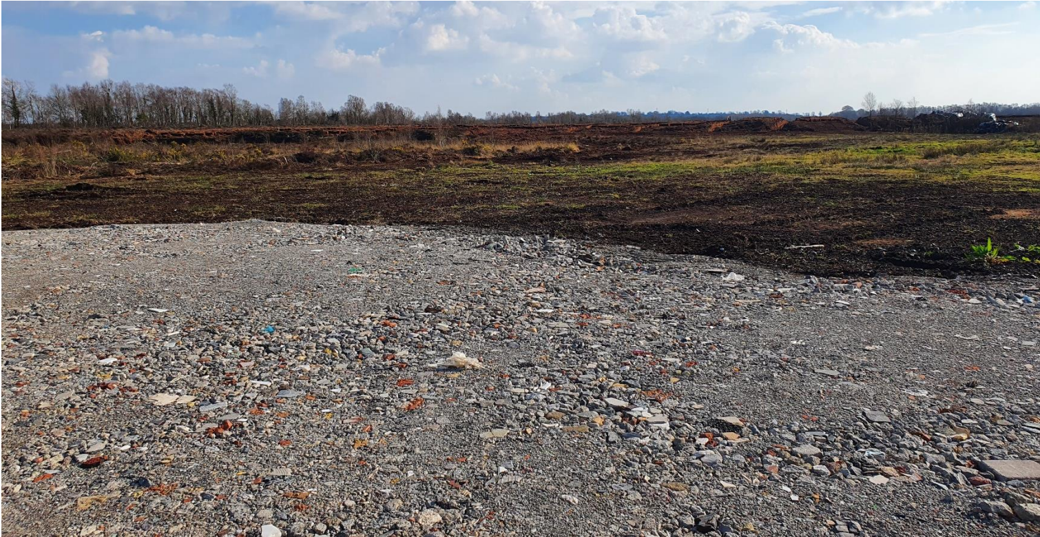
Photo 3: Recently constructed hardstanding with C&D fill noted.
