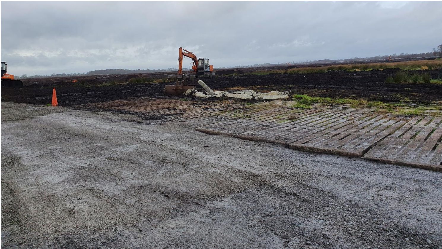
Photo 6: Purpose built roadway at loading area.
