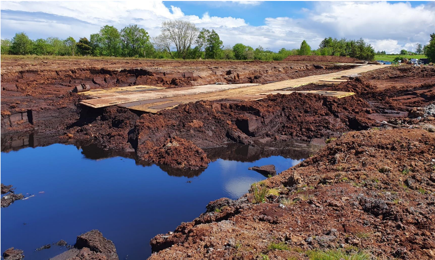
Photo 2: Temporary roadway constructed into excavated area.
