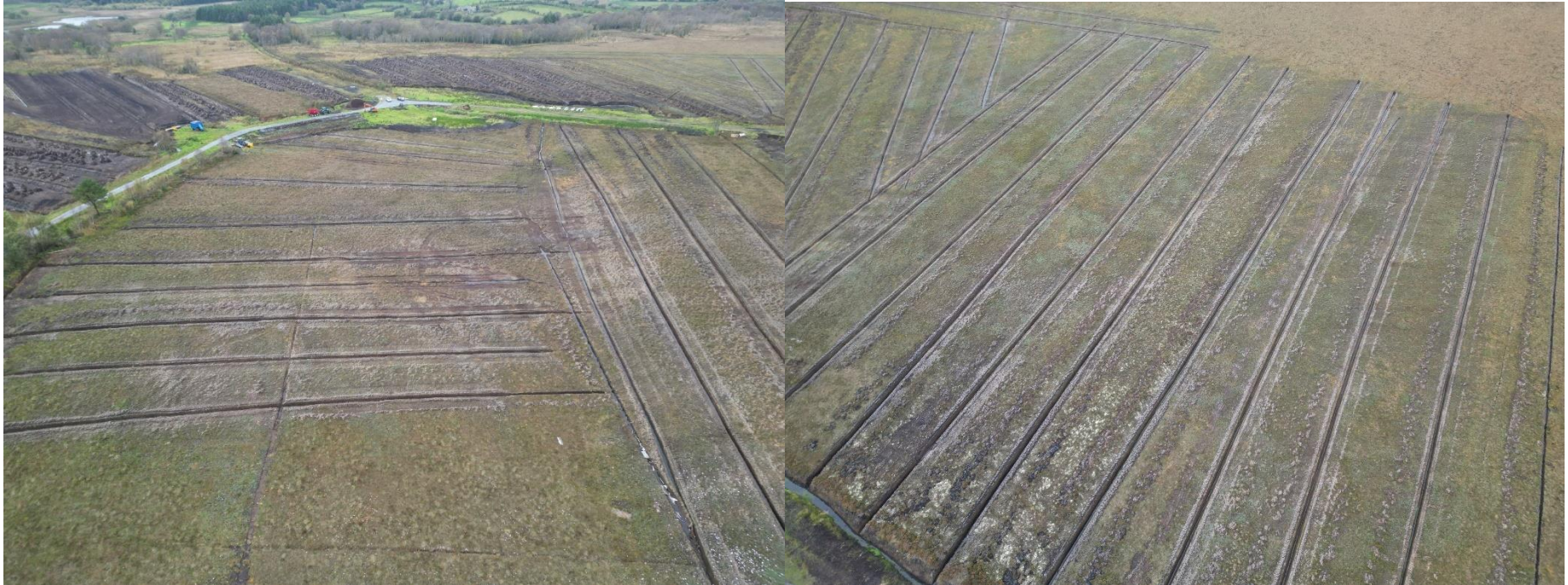
Photos 1 & 2: Preparatory drainage works carried out on the peatland.
