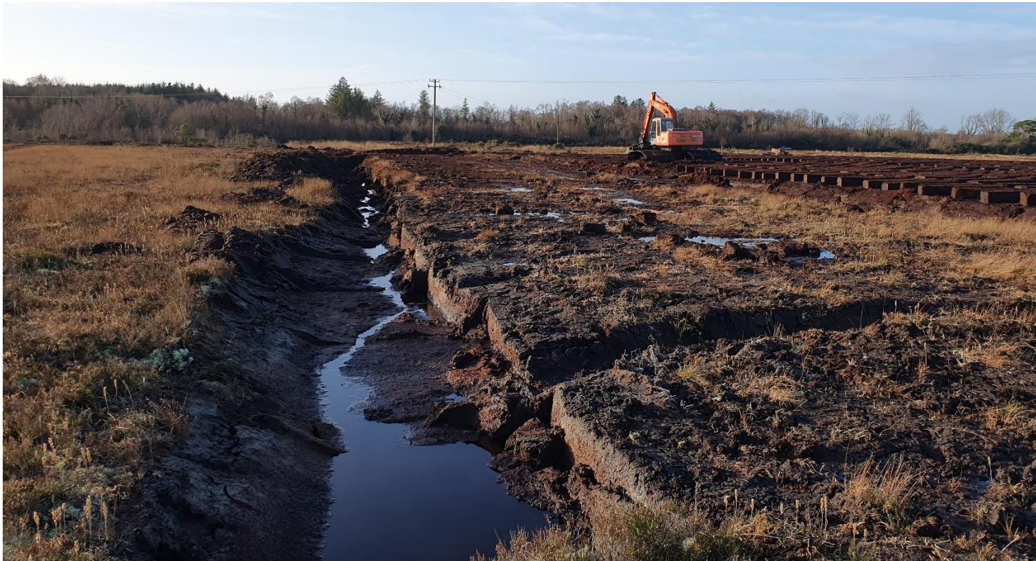
Photo 4: Drainage works in preparation for excavation noted on the peatland.
