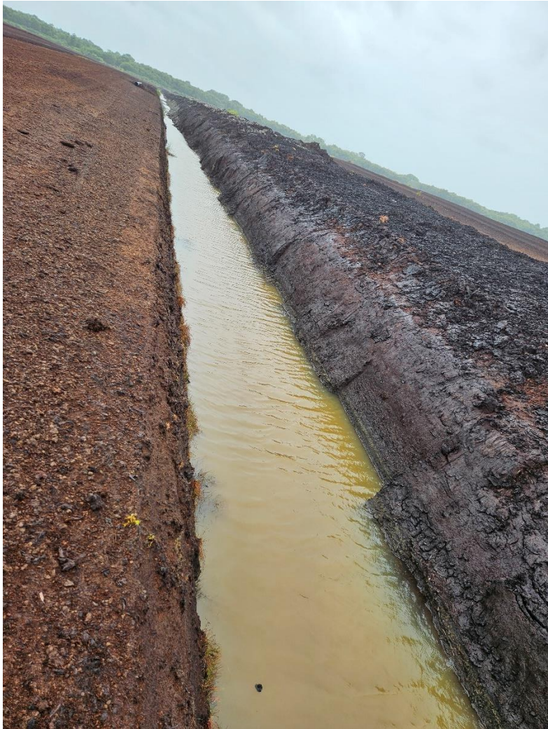
Photos 2 & 3: Milkywhite/brown colour noted in drains on the peatland, also note marl like material close to the surface of the peatland.
