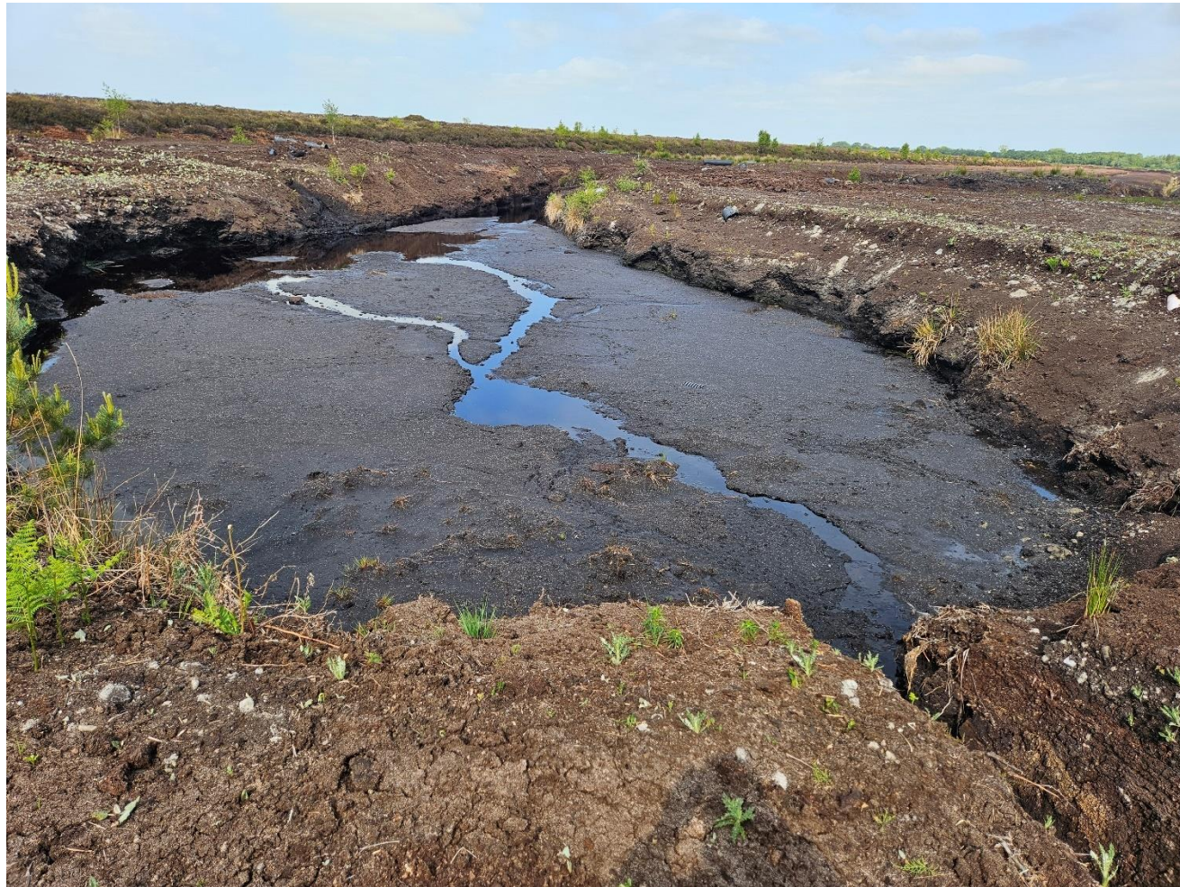
Photo 7: Significant build up of peat noted in one of the sedimentation ponds.
